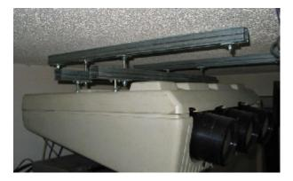
This is an Ampro 4000, which weighs in at 165lbs. Above the ceiling is attic space, so there are 2 more unistrut channels paired with the ones against the ceiling, the hidden struts sit across the top of 3 joists.
