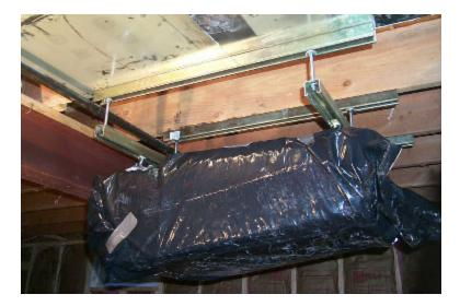
In this example you can more clearly see how the unistrut is attached to the joists above.
